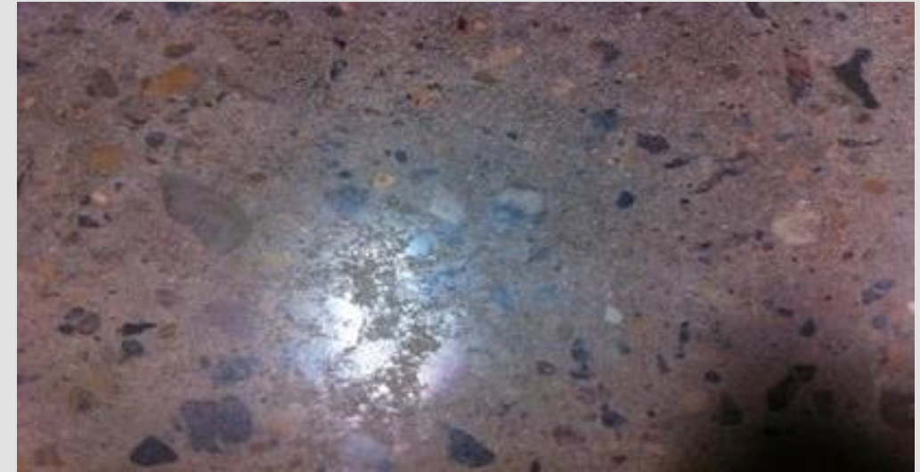
Wear patterns and pitting develop
