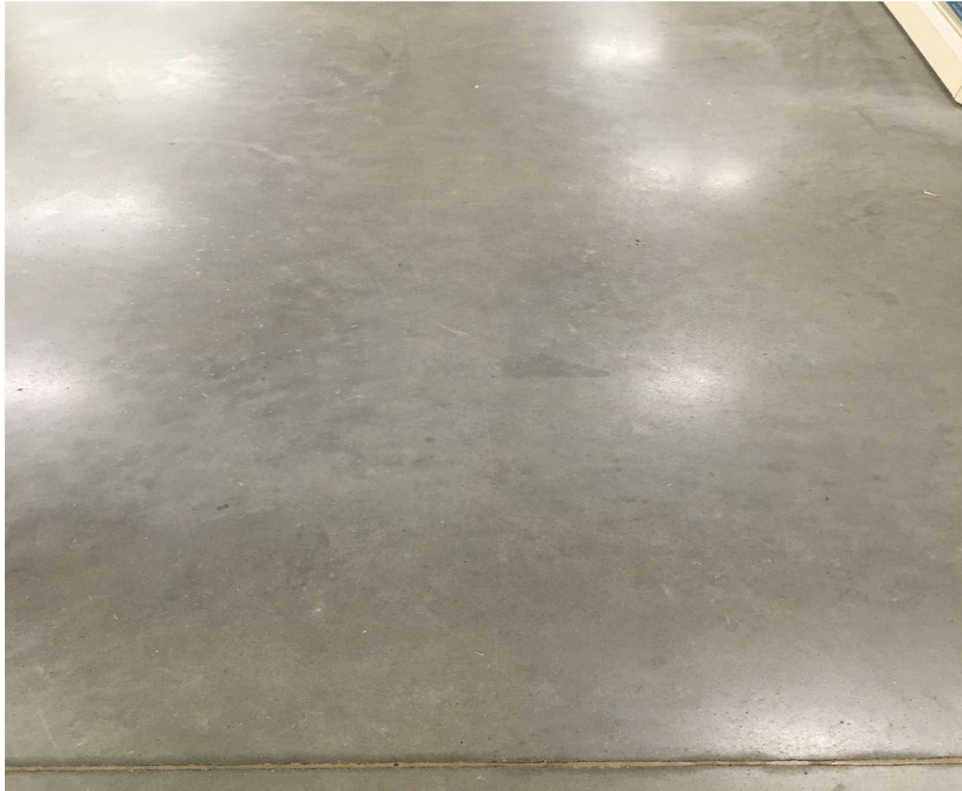
Race Track Wear Aisle Before
